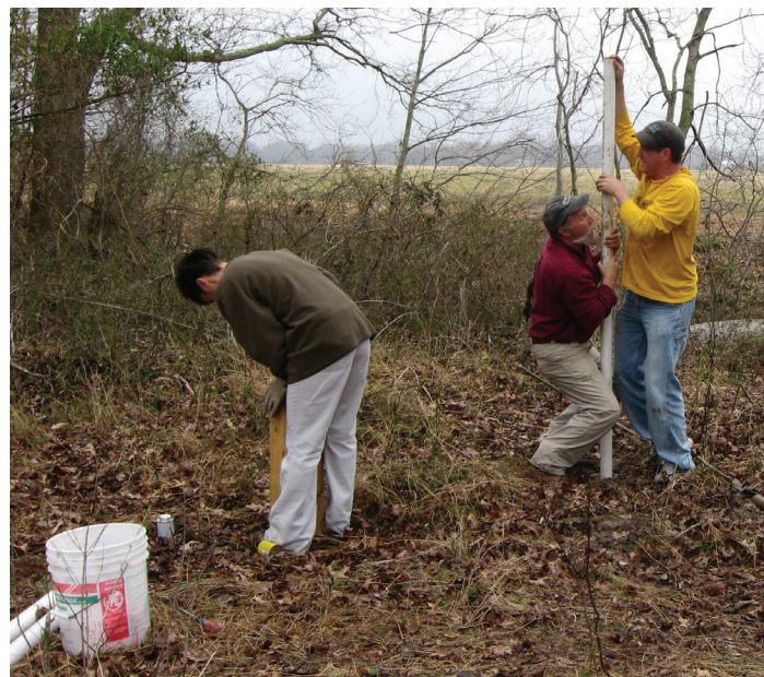
The installation of wells to allow monitoring of groundwater gives information about the concentration of nutrients in the groundwater. Photo by Roman Jesien.
