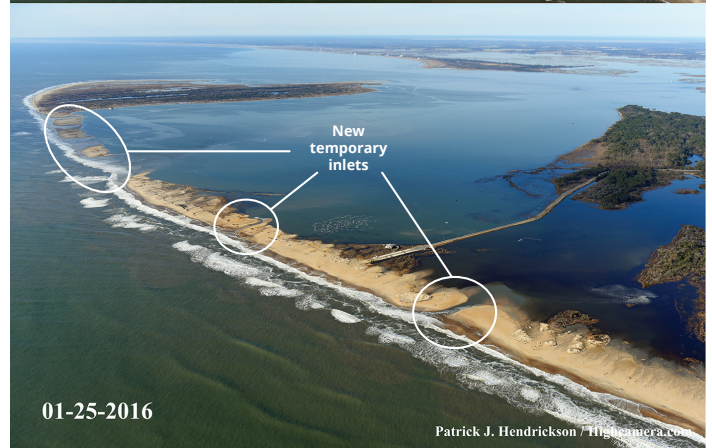
The top photo shows an intact southern end of Assateague Island prior to the blizzard of 22–24 January 2016. That storm breached Assateague Island in several places, as seen in the bottom photo. Photos by Patrick J. Hendrickson/Highcamera.com
